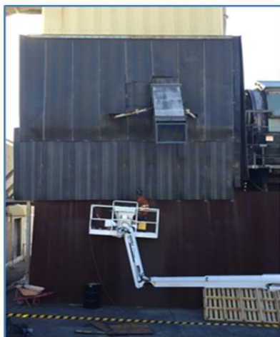
Photo 2 – Completed repairs to transfer house noise curtain, sound barriers around rotary breaker and the new noise attenuated reject chute of the site's rotary breaker.
