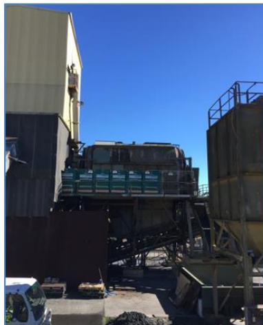
Photo 2 – Completed repairs to transfer house noise curtain, sound barriers around rotary breaker and the new noise attenuated reject chute of the site's rotary breaker.
